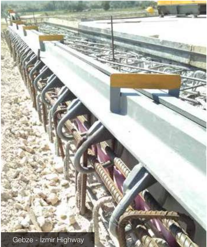
Yavuz Sultan Selim Bridge - Bridge Expansion Joint
